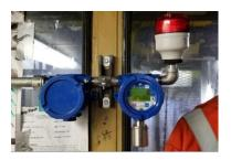
mounting plate for wireless – a true plug and play concept. This method did not affect the existing network and the area previously monitored by the old sensor was covered immediately by RC Systems new wireless gas detectors.
